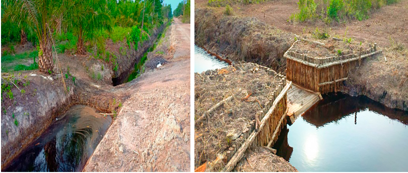
Fig. 3 Different Forms of Canal Blocking Before (left) and After (right) BRGM Intervention (photos by Herman Hidayat, Greg Acciaioli, Massa Djafar, Laely Nur Hidayah, Robert Siburian, Osamu Kozan, and Dicky Rachmawan, July 2019)
