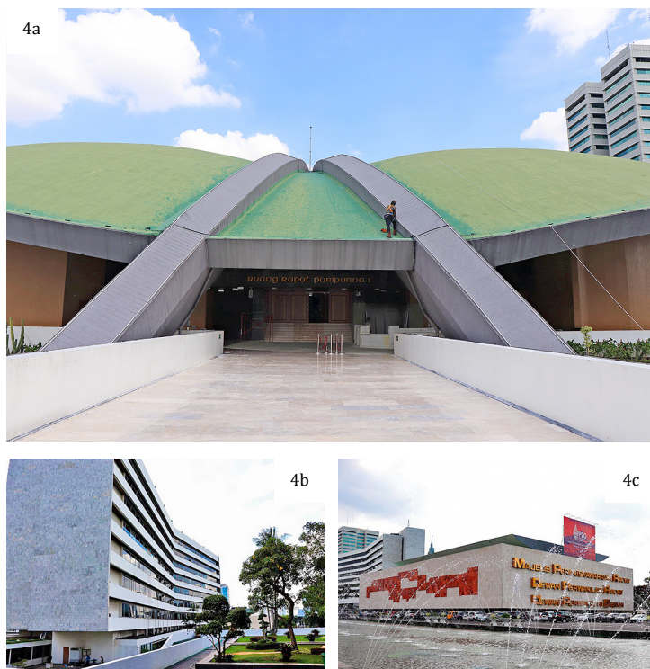
Fig. 4a The Roof Arc Structure of the Nusantara Building
